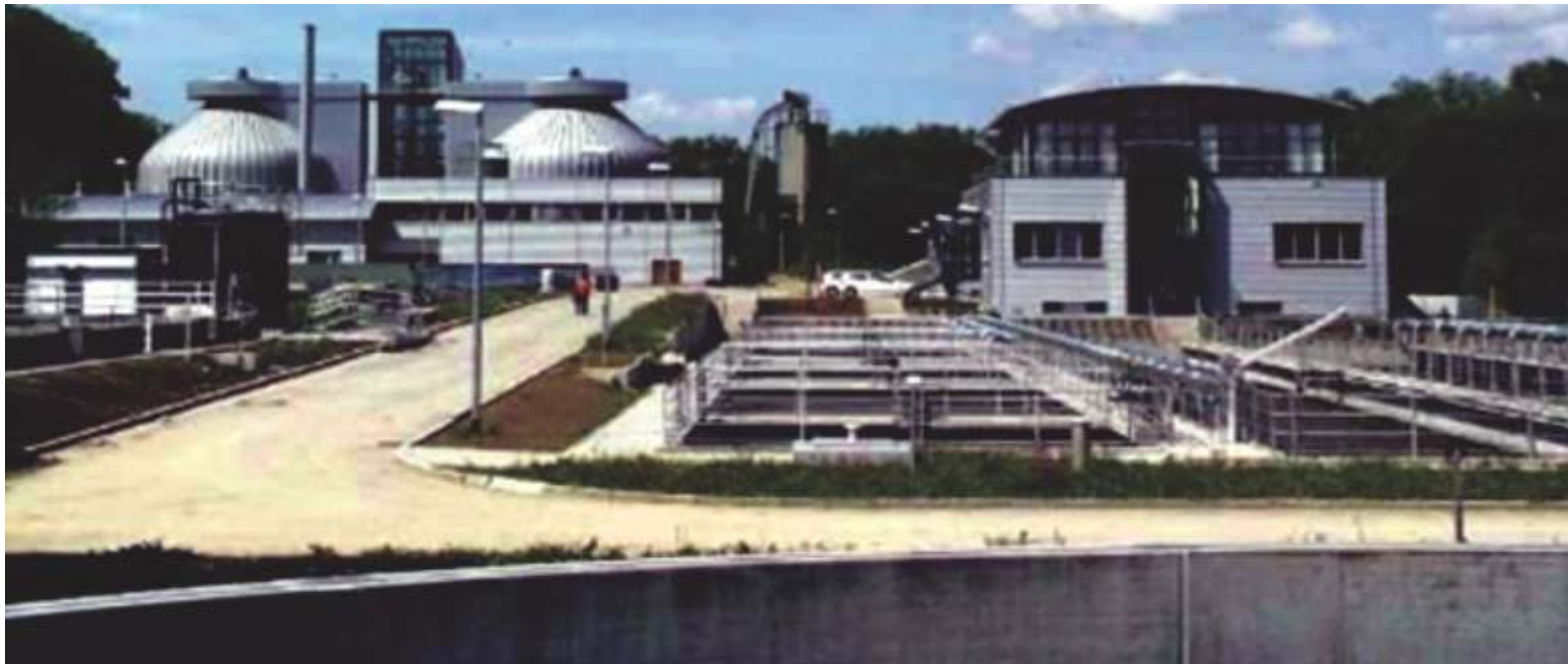
An overview of the waste water treatment plant at Reutlingen in Germany
