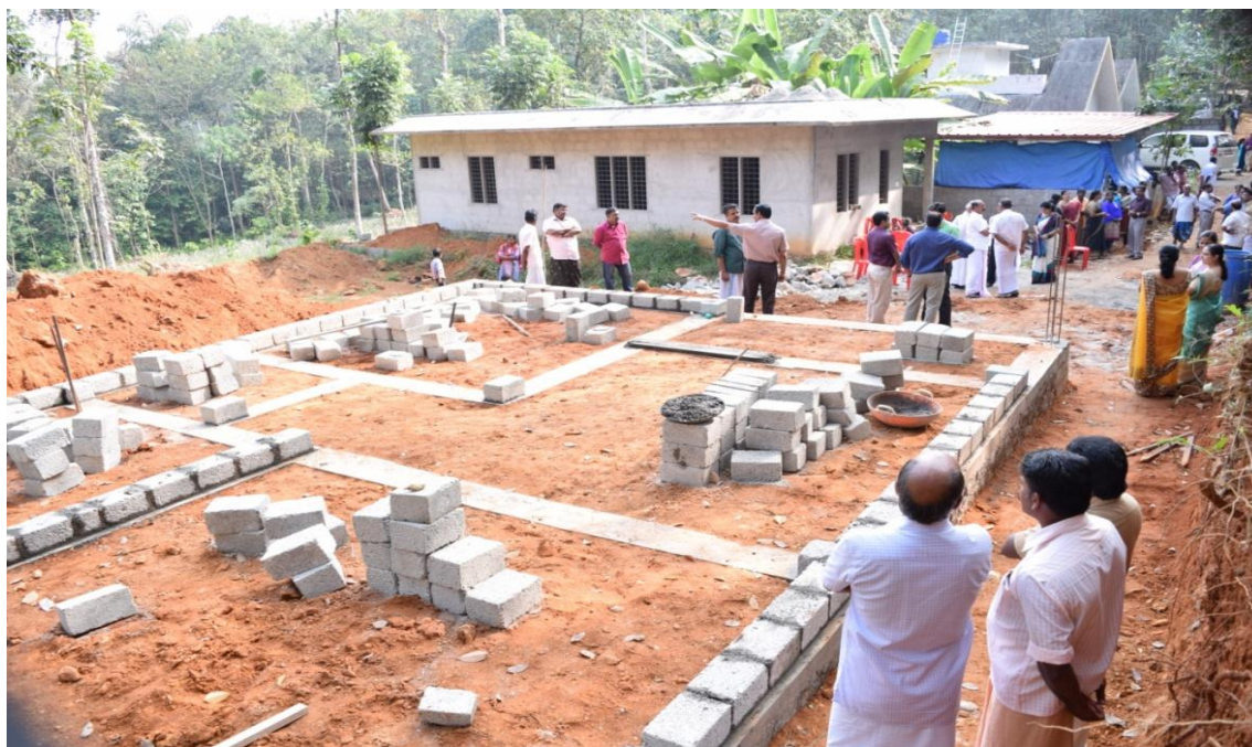
Fig. 9: Swapnaveedu- Laying Plinth belt
