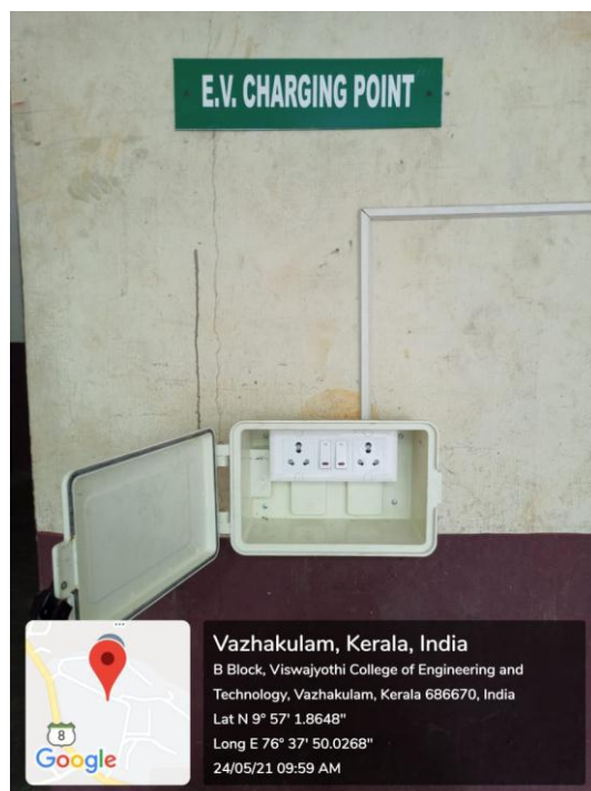
Electric Vehicle Recharging Point for two-wheelers
