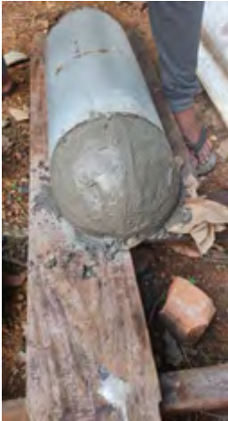
Fig. 4: Moulding using cement
